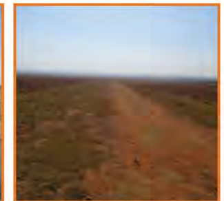
Picture 9: Gravel road covered in vegetation
