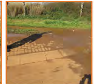
Picture 6: Storm-water crossing above the paved sidewalk
