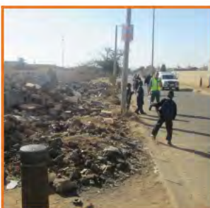
Picture 14: Destroyed multi-purpose centre
