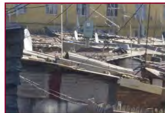
Picture 1 shows congestion and numerous electrical connections.
