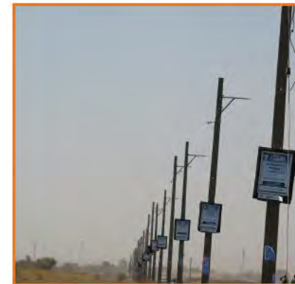
Picture 17: Poles without light fittings
